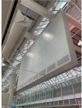
An integrated lift control device allows the display controller and PC to be moved 1.5 metres downwards, as needed, for inspection and maintenance requirements. Additionally, a button for switching off the operating voltage is installed inside this inspection flap.
